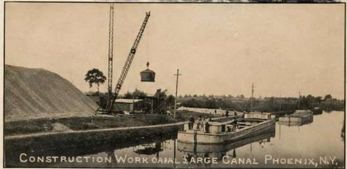
CONSTRUCTION WORK CANAL BARGE CANAL PHOENIX, N.Y. Construction Work on Barge Canal, Phoenix, N.Y. c. 1910
